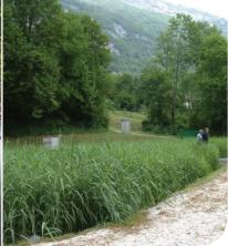
rom their first application as a tertiary treatment, 'final polish', solution through secondary treatment, including nitrification, reed bed wastewater treatment systems are now widely being used for the full treatment of sewage all over the globe through the application of the **Phragmifiltre** system.
