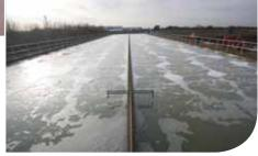
ARM reengineered the distribution and collection system and retrofitted FBA<sup>™</sup> into the existing reed beds. The open water zones were filled with gravel and the gravel depth increased by 500mm. The upgrade works at the Mayfield Farm included the addition/modification of:
