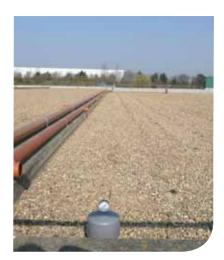
design flow of 40l/s, the wetland cells consisted of open water zones and gravel zones and were planted with *Phragmites australis*. The original system operated passively with oxygen transfer rate of 2.4 - 7.7 g/m<sup>3</sup>/d, removing 4 - 13 g/m<sup>3</sup>/d of COD. This system was unable to treat current volumes of effluent and was failing to achieve compliance.
