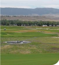
orced Bed Aeration™ (FBA™) is a new wastewater treatment technology which enhances constructed wetland treatment performance. Significantly higher contaminant removal rates are attained along with an increased consistency of performance. Developed in the USA, by our partners Naturally Wallace, FBA™ can be used in both horizontal and vertical flow constructed wetland systems. Blowing air through the wetland system
